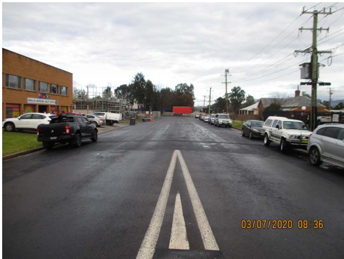
Photo 11 – Rivers Street road formation (viewed from Otho Street intersection)
