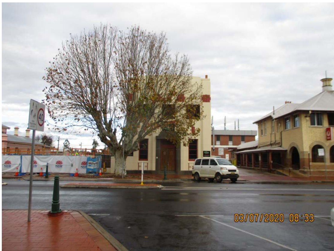
Photo 14 – Two (2) storey building (former Rural Bank) north-west of the development site
