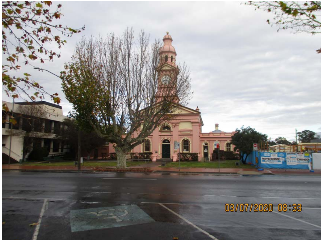
Photo 3 – Inverell Courthouse from Otho Street
