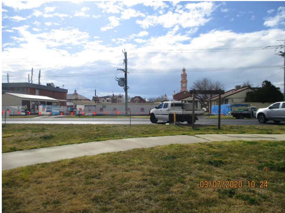
Photo 5 – 2020 (Post-demolition) of one (1) Dwelling (No. 62) in Campbell Street
