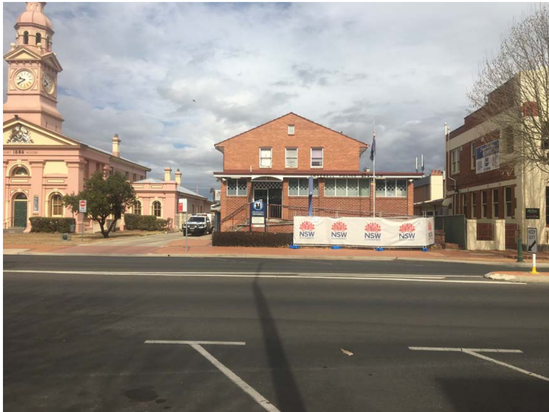
Photo 1 – 2019 (Pre-demolition) Inverell Police Station Site from Otho Street
