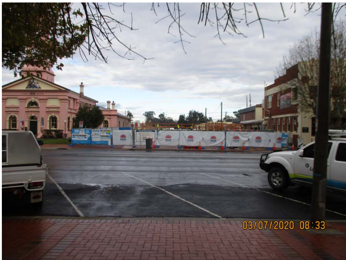
Photo 2 – 2020 (Post-demolition) Inverell Police Station Site from Otho Street
