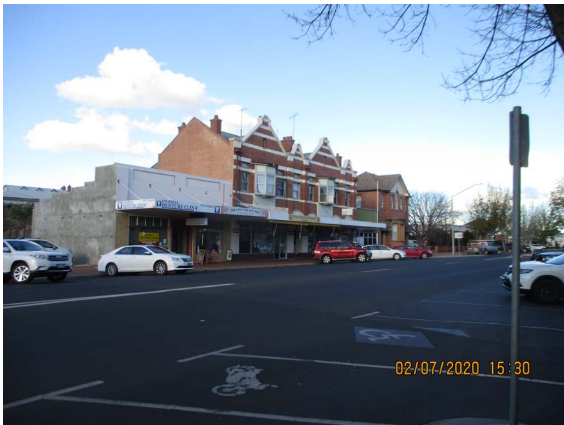
Photo 18 – Two (2) storey commercial buildings in Otho Street opposite the Post Office
